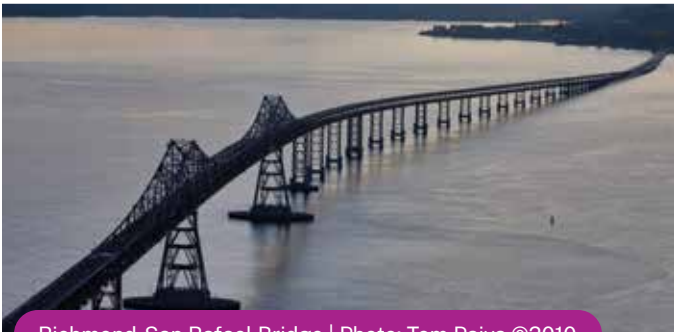
Richmond-San Rafael Bridge | Photo: Tom Paiva ©2010
