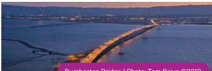
Dumbarton Bridge | Photo: Tom Paiva ©2010
