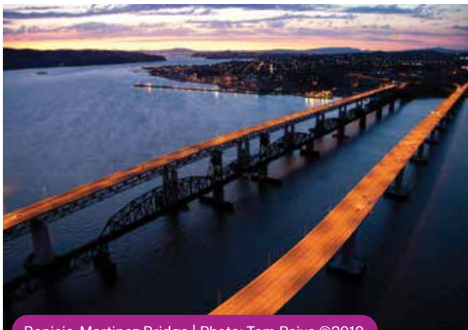
Benicia-Martinez Bridge | Photo: Tom Paiva ©2010
